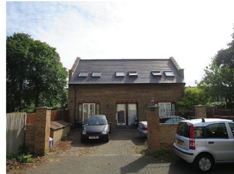
VIEW OF 154A WITH SITE TO THE LEFT
