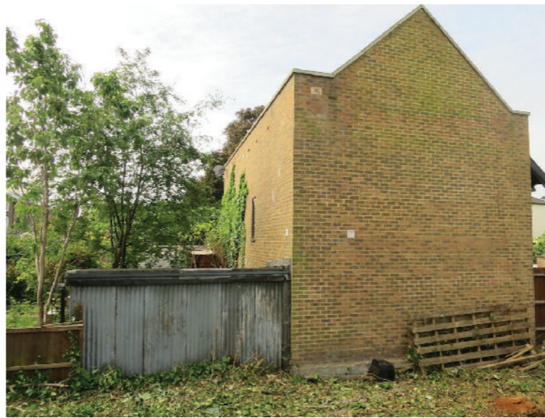
VIEW LOOKING SOUTH AT FLANK WALL OF NO. 154A
